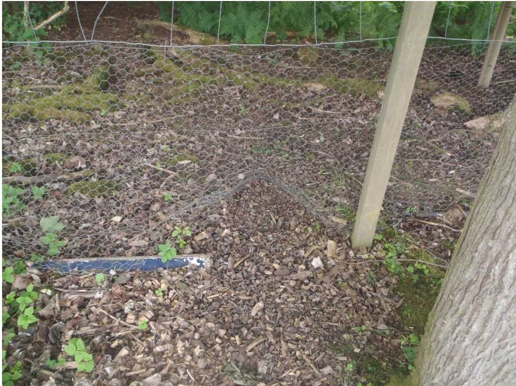
Photograph 4: showing a hole in the boundary fence
